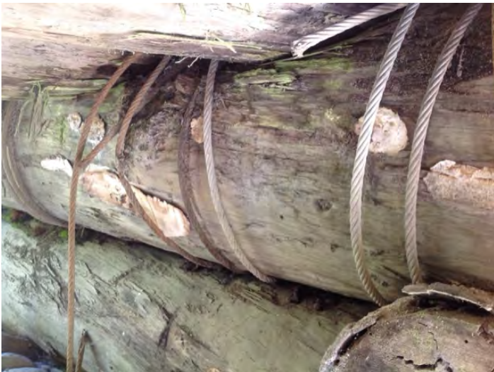
Right Bank Abutment when facing downstream
