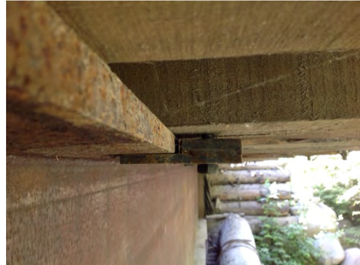
deck clips not correct size but functional for now
