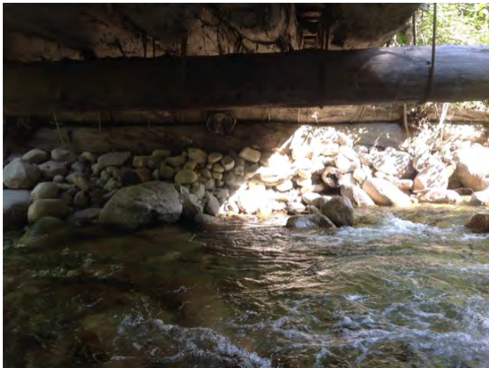
Right Bank Abutment when facing downstream
