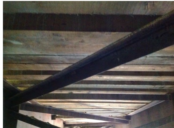
modular panels from underneath
