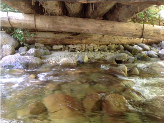
Left Bank Abutment when facing downstream
